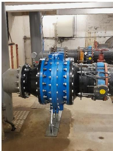
*Intervention by pass kerrouault – nouveau clapet pompe 1 exhaure usine*
